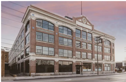
The Assembly today after almost entirely replacing the front façade.
